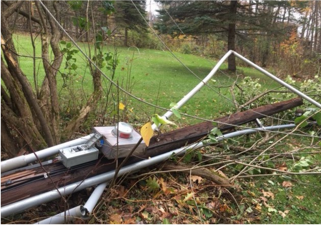
Be prepared for power outages. This pole in Starksboro was blown down during a windstorm in 2017 that took out power for several days.
